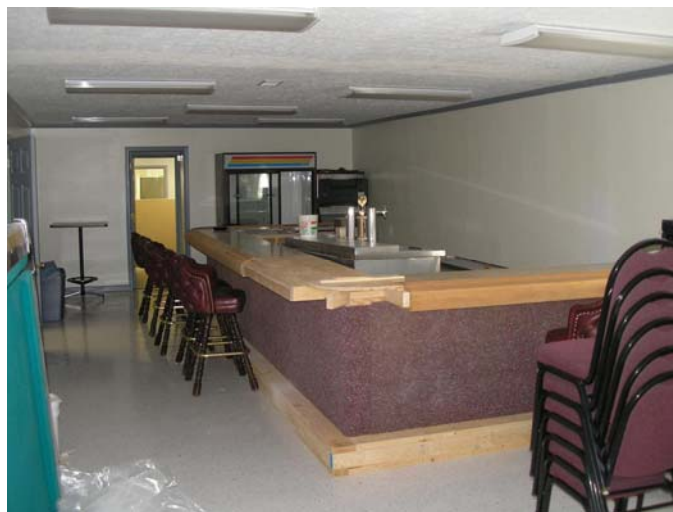
Still Under Construction - Steady progress at POST 604
