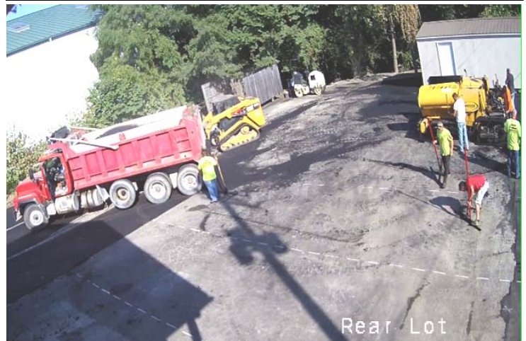
Repaving Parking Lot
