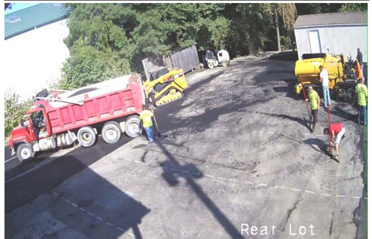
Repaving Parking Lot
